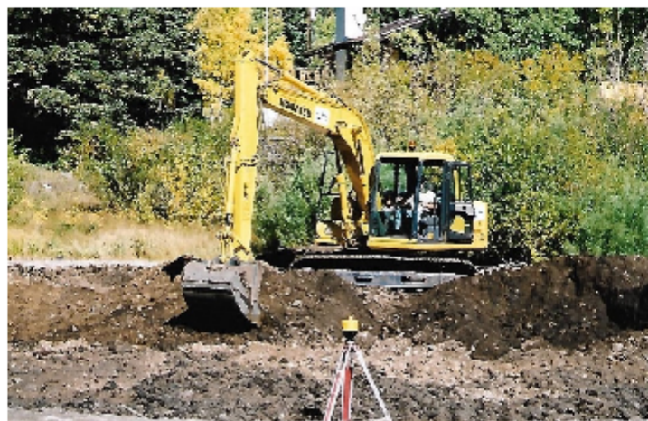
Dredging of lake on west end
